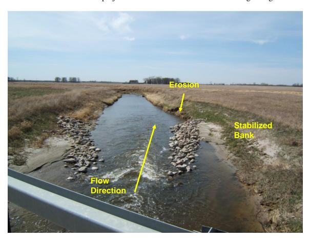
■ Due to the design changes that changed the project's bendway weirs into stream barbs and changed their angles, the final stream barb is actually directing flow directly into the opposite bank instead of down the middle of the channel and is creating a new erosion problem.
